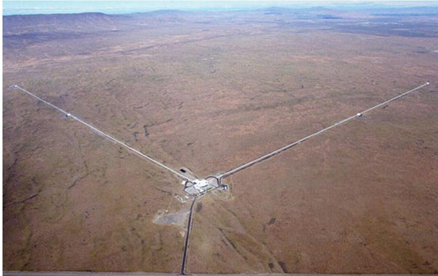
**LIGO's antennas are L-shaped, with perpendicular arms 2.5 miles long. Inside each arm, cocooned in layers of steel and concrete, runs the world's largest bottle of nothing, a vacuum chamber a couple of feet wide containing 2.5 million gallons of empty space. At the end of each arm are mirrors hanging by glass threads, isolated from the bumps and shrieks of the environment better than any Rolls-Royce ever conceived.**
